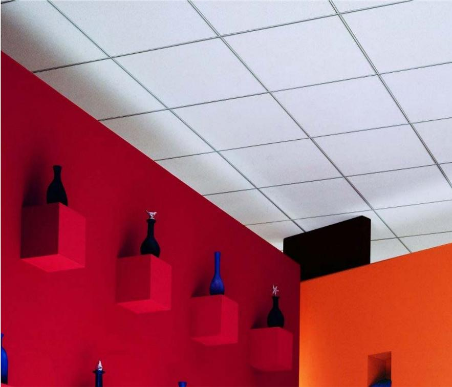
With micro perforations that provide a smoother look and good sound absorption, these panels offer upscale appearance at a mid-range price. Olympia™ Micro™ Acoustical Panels offer high level light reflectance, mold and mildew resistance, ceiling attenuation and noise absorption, making them a perfect choice for classrooms, hotels, reception and lobby areas, restaurants and retail stores.
