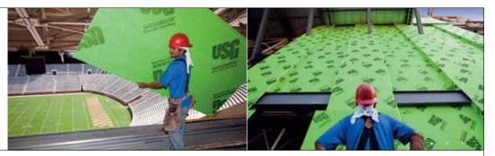
"At one point the whole west side of the stadium was exposed with SECUROCK glass-mat sheathing, but since we knew the product could get damp, we knew we were protected," explained Layton. "We also sealed up other parts of the stadium with SECUROCK so we could continue to work inside and didn't have to worry about the weather affecting us. That helped push the schedule along."
