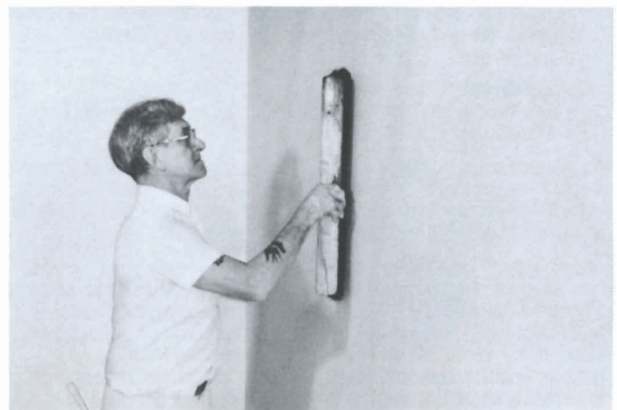
Basecoat surface is left rough and open for finish coat application.
