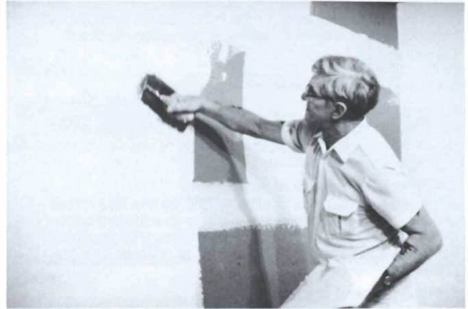
Application of DIAMOND Veneer Basecoat Plaster over IMPERIAL Gypsum Base.
