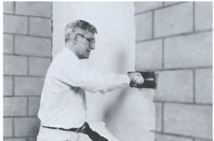
Application of DIAMOND Veneer Basecoat Plaster over masonry or monolithic concrete treated with a bonding agent .
