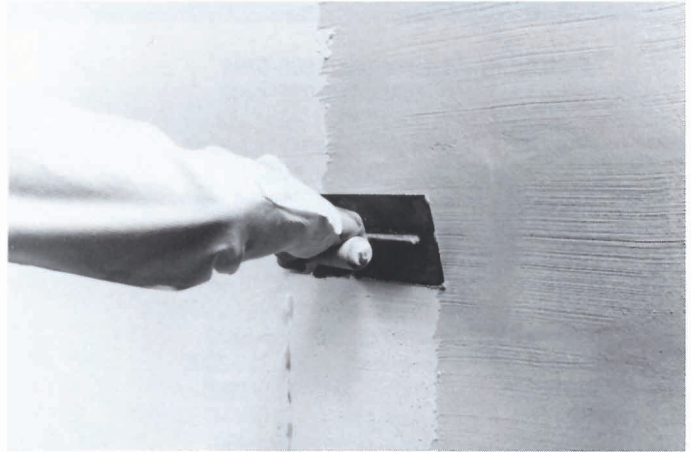
Smooth trowel finish coat applied over DIAMOND Veneer Basecoat Plaster.
