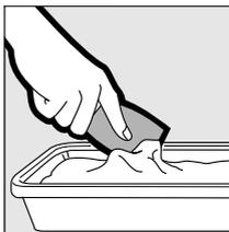
Keep the blade clean, especially of dried bits of compound, to avoid leaving scratches in the wet joint compound as you draw the knife over it. Discard any compound containing dried bits of material. Clean blade by drawing it over edge of pan.
