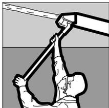
The box is controlled with specially designed handles available in various lengths (including long handles suitable for working overhead on ceiling joints). As you apply pressure to the box handle, compound is pushed onto the wall. The lever on the handle end will lock the box at the desired angle. The box may also have an adjustment wheel to control the amount of crown left by the box; you may need to experiment with the adjustment wheel to find the optimum setting for a particular task.
