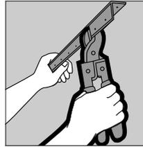
When pushing the bead onto the corner, be careful that the flanges do not spread beyond a 90° angle; this will make it hard to cover them with joint compound.
