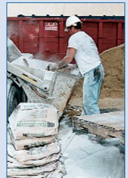
Bags of gypsum concrete underlayment were mixed with sand and water to create a slurry.
