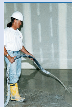
The gypsum underlayment mix was pumped via hoses and poured directly onto the floor.
