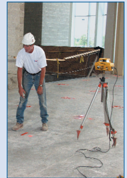
Barrier Corp. flooring applicator crews used a laser to measure existing floor elevations.
