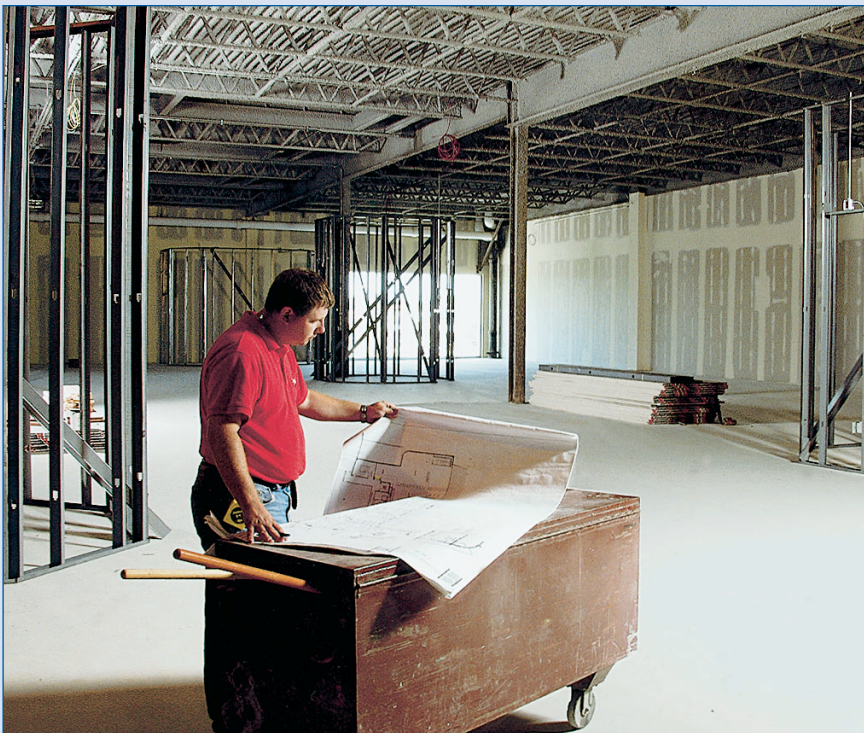
Skip Pastore, site manager for Barrier Corp., reviews construction plans following application of the gypsum concrete underlayment floor. The floor is ready for continued trade traffic within 24 hours.
