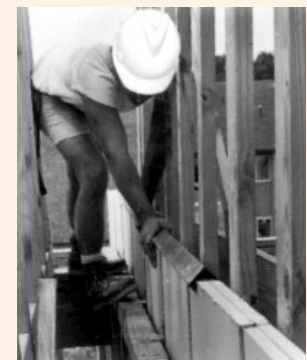
Steel C-runner fits over the studs and panels. A second C-runner is then screw-attached back to back to lower the runner to hold the next level of studs and liner panels.
