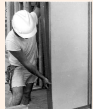
Steel H-stud slides in place over gypsum liner panels.
