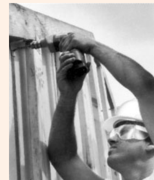
An aluminum breakaway clip is screw-attached to studs and framing. Under fire exposure, the clips break away, permitting the fire-damaged wall to fail while leaving the separation wall intact.
