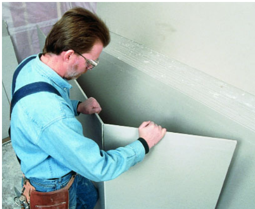
Gypsum board scores extremely high on nearly all sustainable design criteria. It is made from an abundant and non-endangered mineral (gypsum) and has low embodied energy. Drywall made from recycled gypsum reduces landfill waste resulting from fossil-fuel power plant generators.
