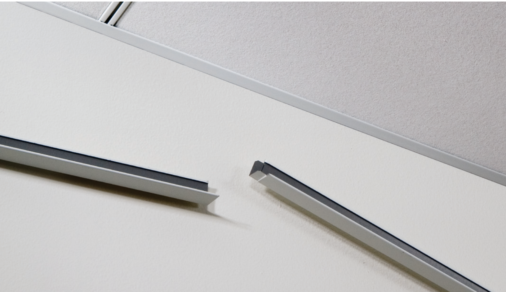
DOWN M7 Overlapping Wall Angle
