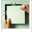
Measure and cut out new drywall panel section to fit damaged area. Screw through new drywall into each drywall repair clip. Screw into drywall; position screw opposite screw holding clip and about 3/4" from edge. Remove tabs from each drywall repair clip.
