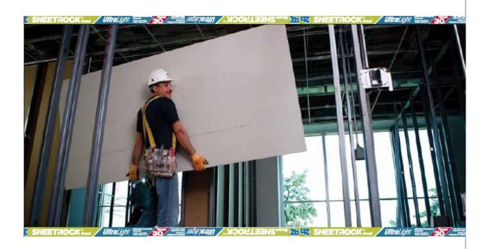
SHEETROCK® UltraLight FIRECODE® 30 Panels have been formulated to achieve comparable strength and performance characteristics of standard 5/8" SHEETROCK® FIRECODE® Core panels at a significantly reduced weight. The panels feature an engineered core encased in proprietary 100% recycled face and back papers for a high strength-to-weight ratio composite design.
