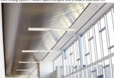
"We proposed several Curvatura layouts until we arrived at an elegant Swoosh like curve to fit within the bulkheads, covering electrical and mechanical components at various elevations. Even with direct sunlight, the Curvatura ceiling finish looks uniform and compliments the overall space well."
