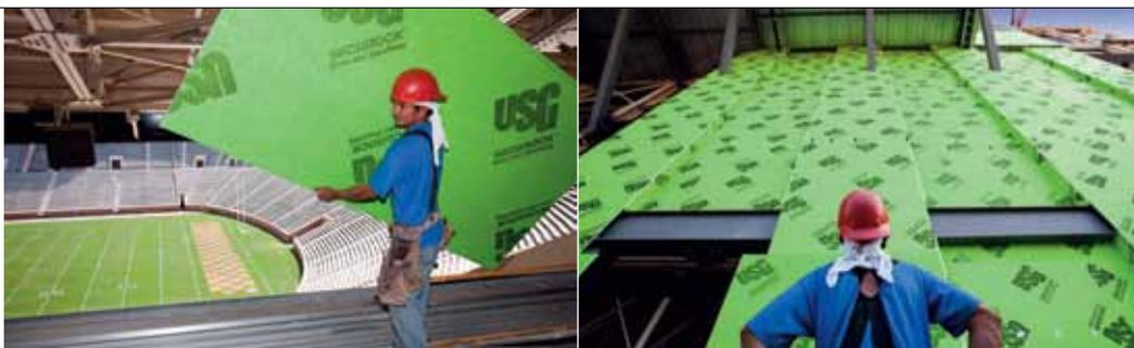
“At one point the whole west side of the stadium was exposed with SECUROCK glass-mat sheathing, but since we knew the product could get damp, we knew we were protected,” explained Layton. “We also sealed up other parts of the stadium with SECUROCK so we could continue to work inside and didn’t have to worry about the weather affecting us. That helped push the schedule along.”
