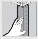
Method 2 — USG Sheetrock\* Brand Paper-Faced Metal Corner Bead and Trim Measure length of corner and cut trim to length with metal snips. For vertical wall installations, cut the corner trim 1/2" (12.7 mm) shorter than the wall height.
