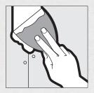
Center and lightly press tape into wet joint compound with fingers. Draw 5" knife firmly along joint to tightly embed tape. Be sure there is sufficient joint compound under tape to prevent blistering of the tape.
