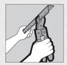
Force bead onto corner being careful that the flanges don't spread beyond 90° angle, making it hard to cover them with joint compound.
