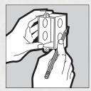
Cut with keyhole saw, jab saw or rotozip. Wear a dust mask if excessive dust is produced and the area cannot be ventilated.
