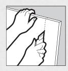
To break the panel core, securely grasp the board edges on both sides of the score line and snap board with a quick, firm movement.
