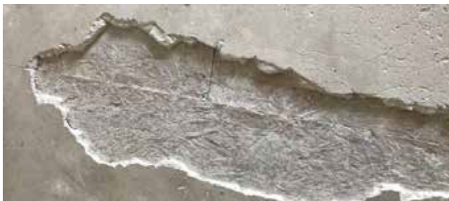
A UL Classified and specified repair product such as USG Durock™ Tuf-Skim™ Floor Patch is required to keep the fire rating of this floor.
