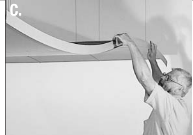
Install the Edge Trim by sliding each trim segment onto the grid. For ease of installation, Edge Trim segments are designed to be about 1/2-inch shorter than the Main Tee segments.
