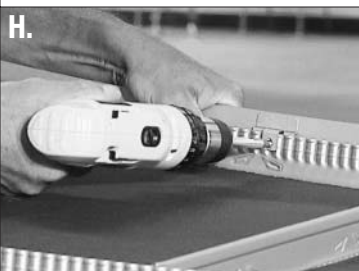
Squeeze the trim against the grid to ensure a proper fit. Then, screw-attach the trim segments to the grid with number-six by three-eighths self-tapping screws. Be sure to install at least two screws per trim segment.
