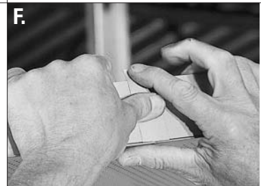
Hook the tab over the bottom edge of the trim. Then, bend over the top of the splice as shown here. It's easiest to install Fascia Splices progressively.
