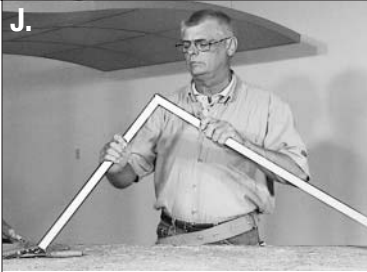
The finished field-cut Main Tee with the cross Tee installed should look like this.
