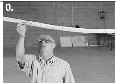
Next, examine the profile of the completed row from the side. The curve of one tee should flow smoothly into the curve of the next. If the curves are not flowing smoothly, adjust the hanger elevations either up or down.
