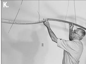
Continue installing Main Tee segments. Refer to the Ribbon Drawing to select each tee.
