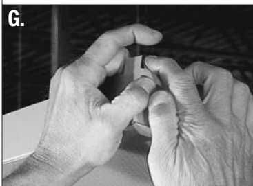
Next, apply Corner Caps. Hook each Corner Cap over the bottom edge of the trim, then bend over the top as shown here.
