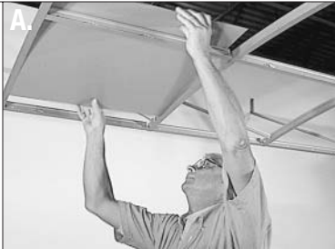
A. Lay CURVATURA 2'x2' panels into the grid one at a time.
