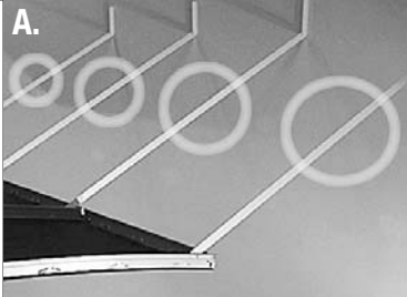
Remove any temporary bracing.
