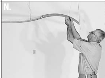
The accuracy of the first row of Main Tees will ultimately determine the quality of the installation so be sure to check the integrity of the completed row. Extra care at this point will prevent alignment problems in the rest of the installation.
