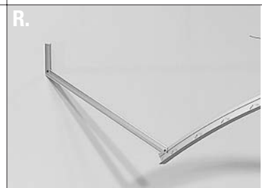
It's important that the first row of Main Tees remains stable during the entire process. As a final step, install temporary bracing to the ceiling or walls, as each row is completed to ensure that it remains straight and rigid.
