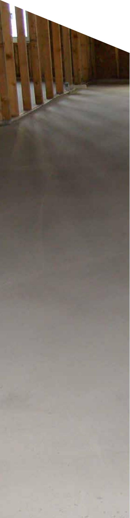
The exceptions to the drying times previously listed are the USG Durock™ Quik-Top™ Self-Leveling Underlayment Series of products. These products have a unique drying technology that allows for floor covering installation 15 hours after underlayment installation.
