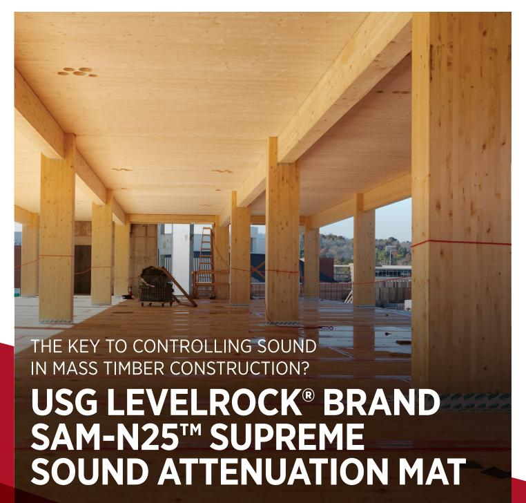
Mass timber construction provides a beautiful and more sustainable alternative to steel and concrete framing. The challenge is that wood transmits sounds more easily than concrete or steel, making it difficult to meet strict STC and IIC sound code requirements.
