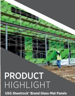
Mold Tough\* — High performance interior panels create moisture- and mold-resistant walls and ceilings. Panels are engineered to be moisture and mold resistant in interior pre-rock applications, feature warranted weather exposure performance, an inorganic face and back, include a tapered edge and accept the application of USG finishing systems.
